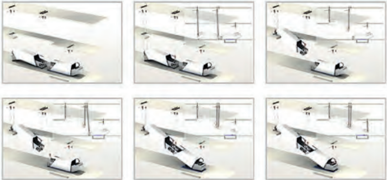
Figure 8.3 Installation in sections is useful when the roof of the building can not be removed
