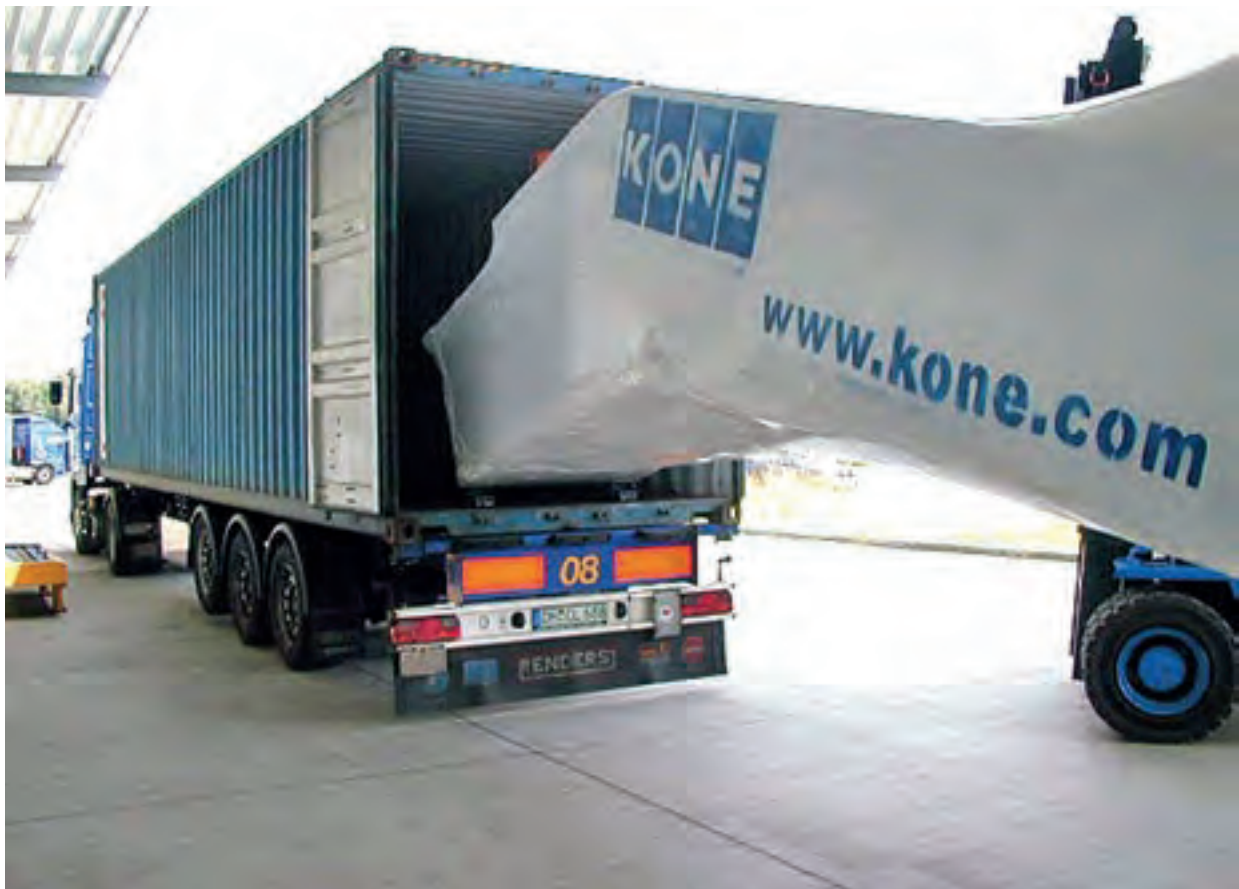
Figure 7.7 Unloading an escalator using forklift trucks
