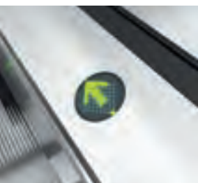
LED traffic lights located in the decking
